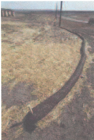
A compost filter berm permanently stabilizing a hillside.
