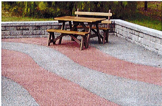
← Figure 7: POROUS CONCRETE
