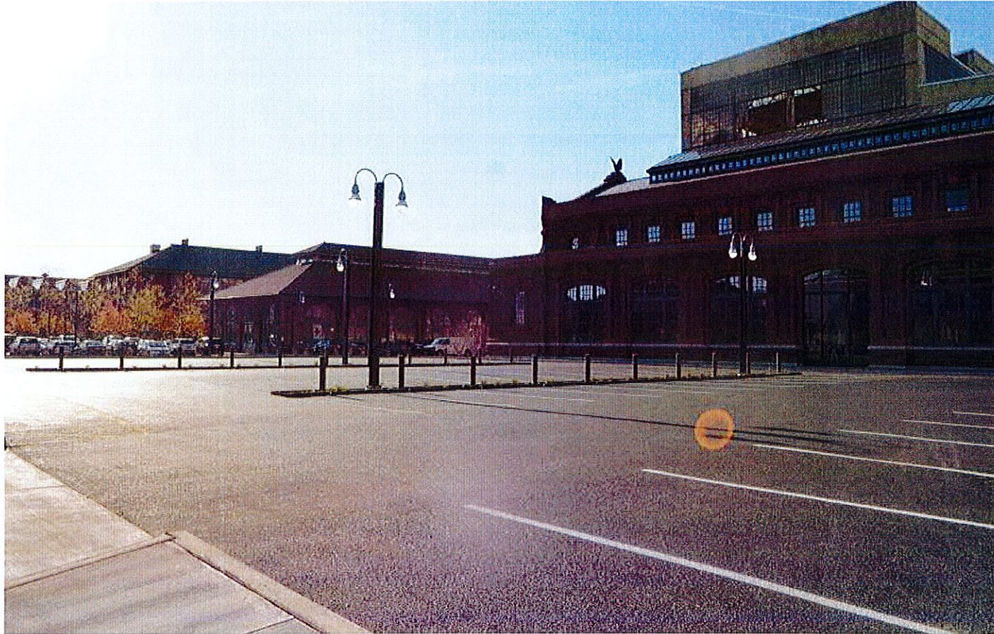
Figure 17: URBAN OUTFITTERS (NAVAL YARD BLDG 18) NORTHEAST POROUS PAVEMENT FINAL
