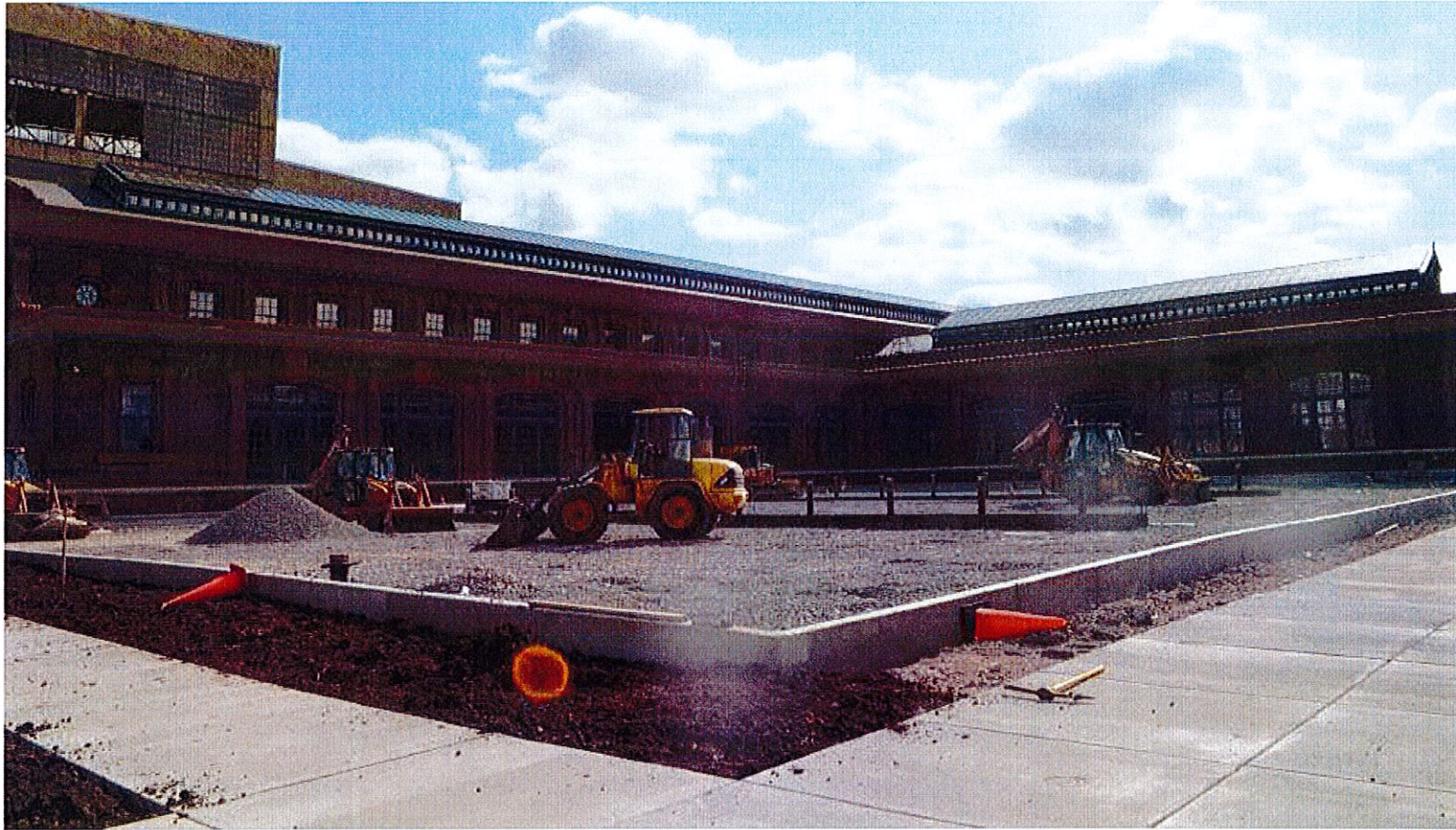
Figure 16: URBAN OUTFITTERS (NAVAL YARD BLDG 18) NORTHEAST PARKING LOT BASIN CONSTRUCTION
