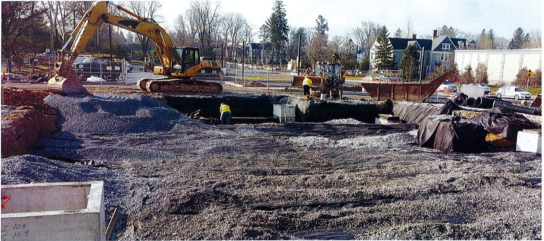
Figure 25: DEVON YARD POROUS PAVEMENT SEMI-FINE AGGREGATE LAYER
