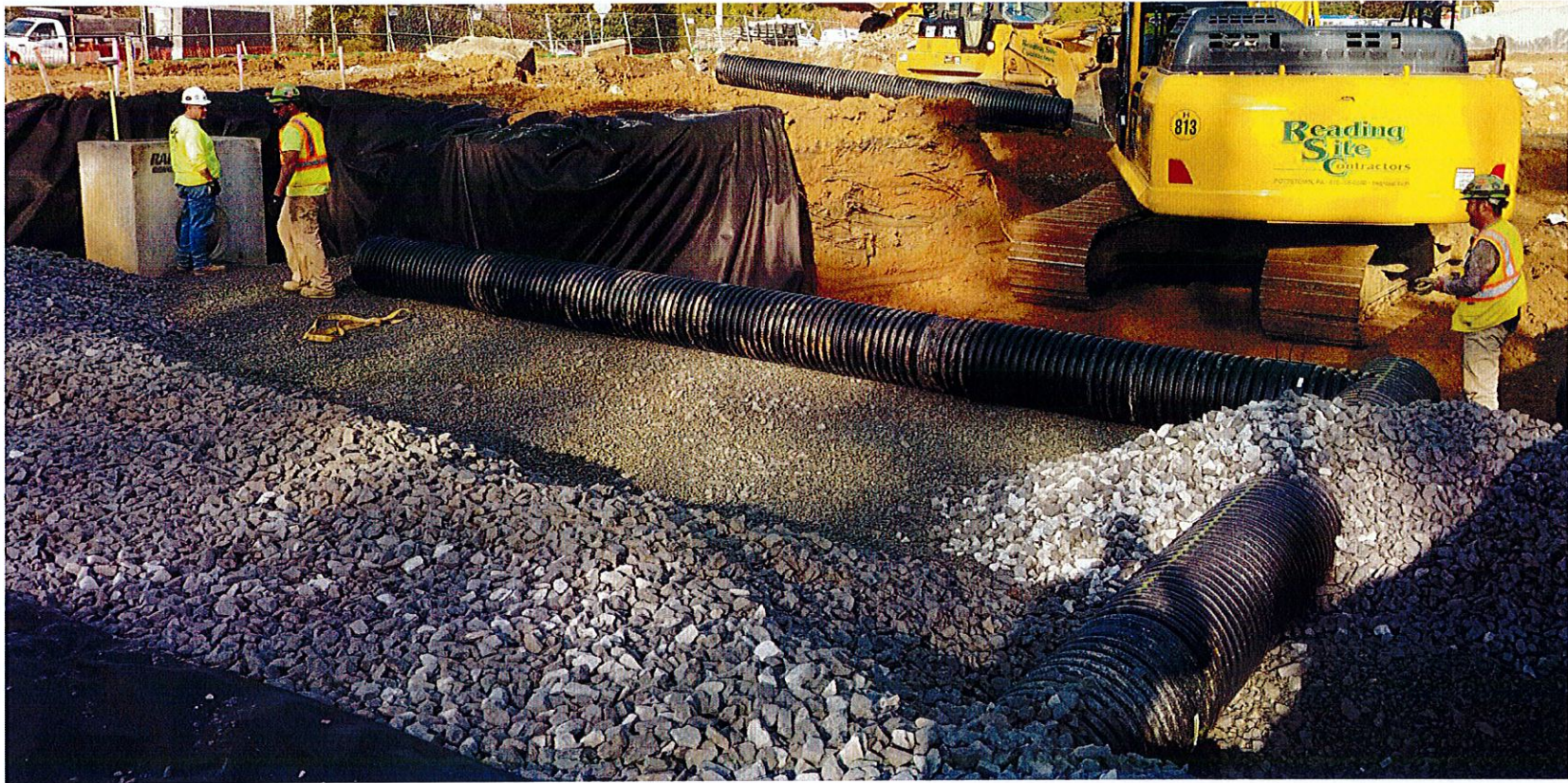
Figure 27: DEVON YARD POROUS PAVEMENT BASIN 3 CONSTRUCTION
