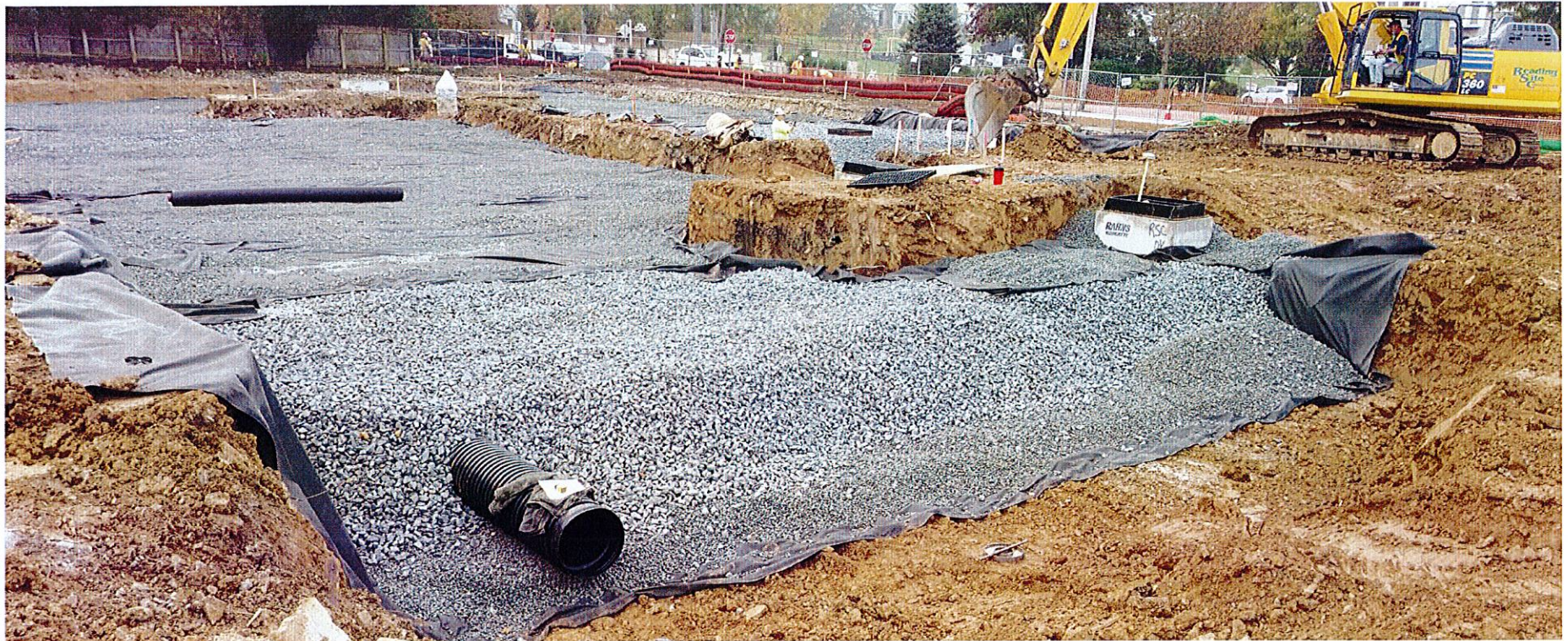
Figure 24: POROUS PAVEMENT LARGE AGGREGATE LAYER COVERING CORRIGATED PIPE PLACEMENT
