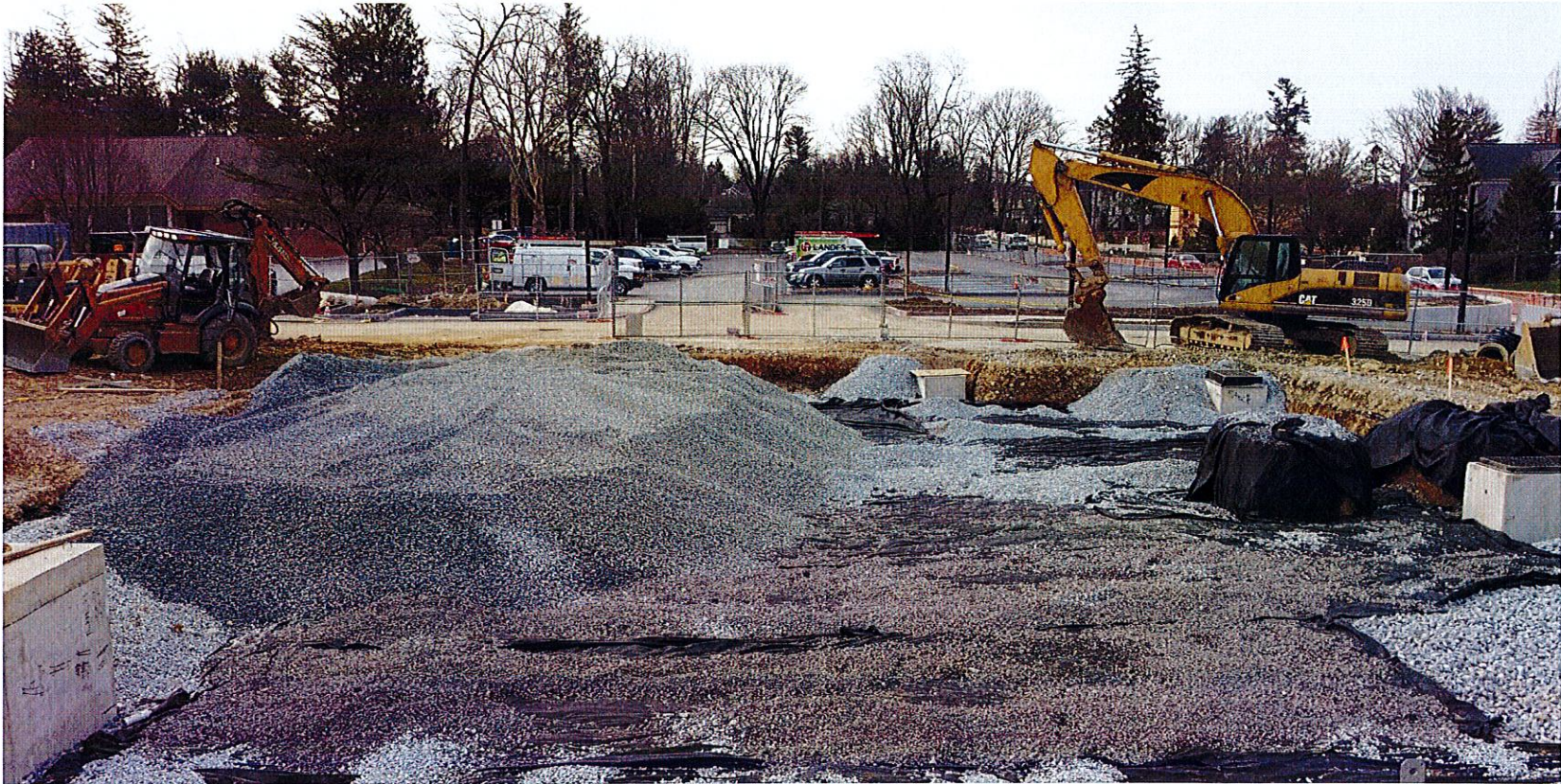
Figure 26: DEVON YARD POROUS PAVEMENT CHOKER COURSE
