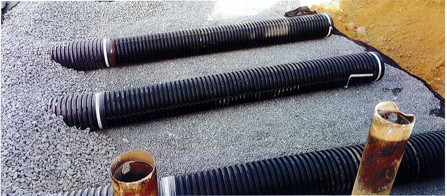
Figure 23: DEVON YARD POROUS PAVEMENT CORRIGATED PIPE PLACEMENT
